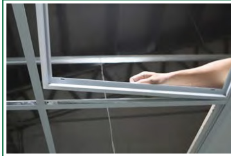
Step 2 - Insert the Conversion Box Frame into the ceiling grid.
