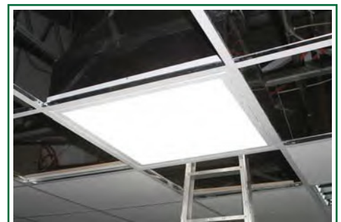
Step 12 - The finished result should look like this. You can now put the surrounding ceiling panels back in place.
