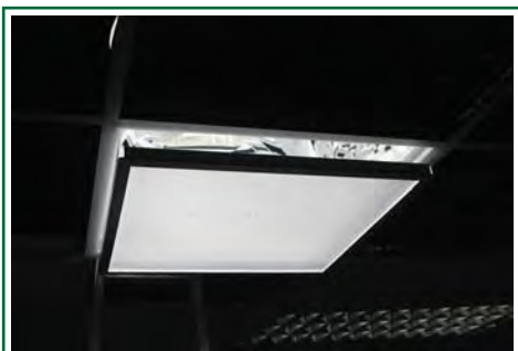
Step 10 - Repeat this for all four springs. Once done the Diffuser Holder should hang approx 50mm below the Conversion Box.
